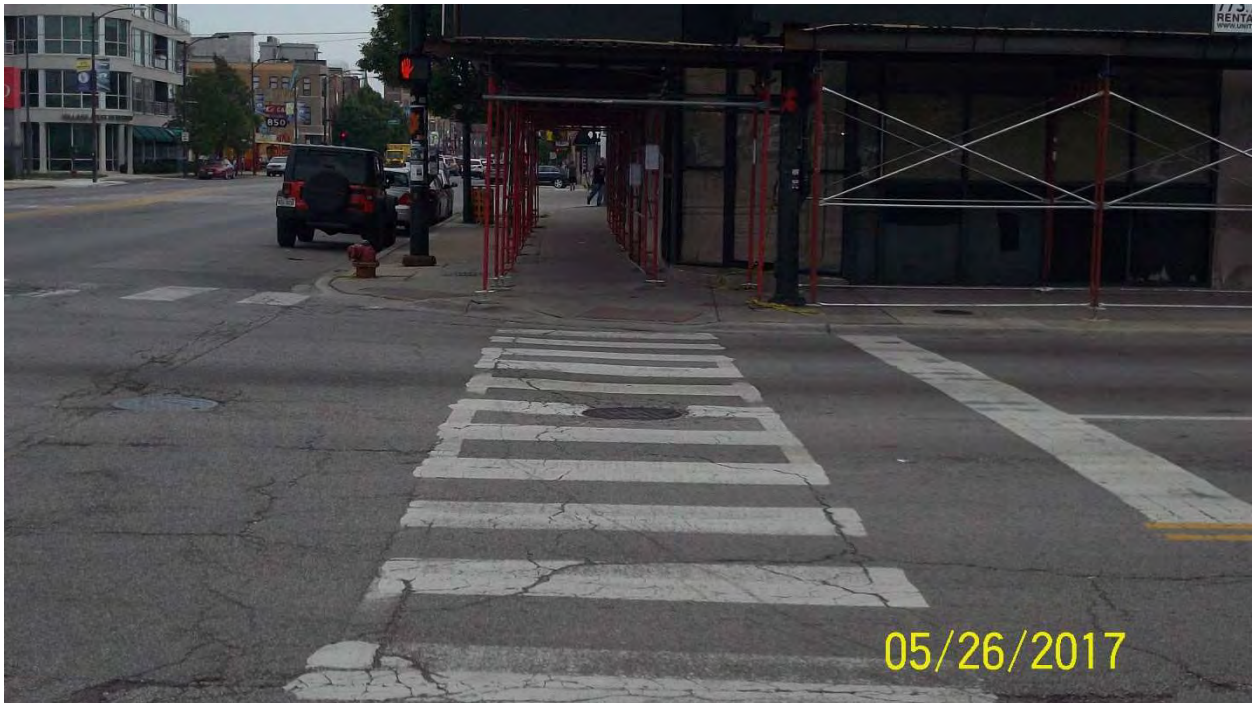
Photo 16: Southeast corner of Chicago Ave. / Western Ave. – Looking North
