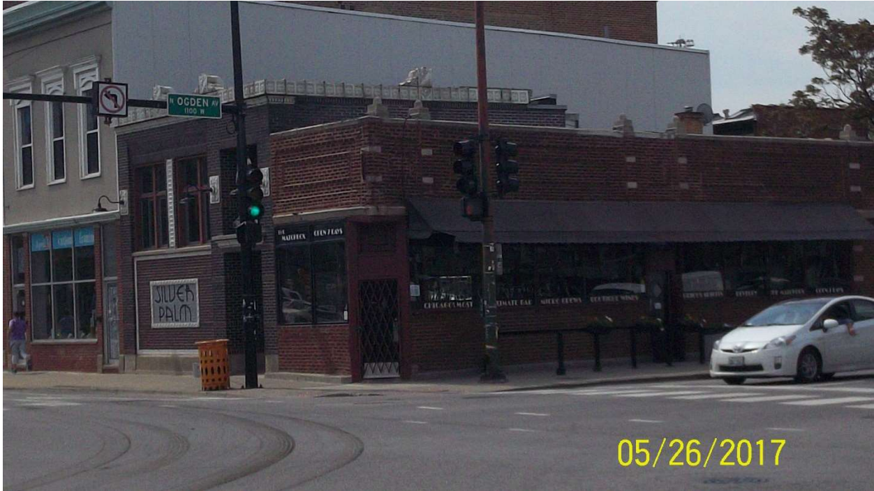
Photo 51: North corner of Milwaukee Ave. / Ogden Ave. – Looking South
