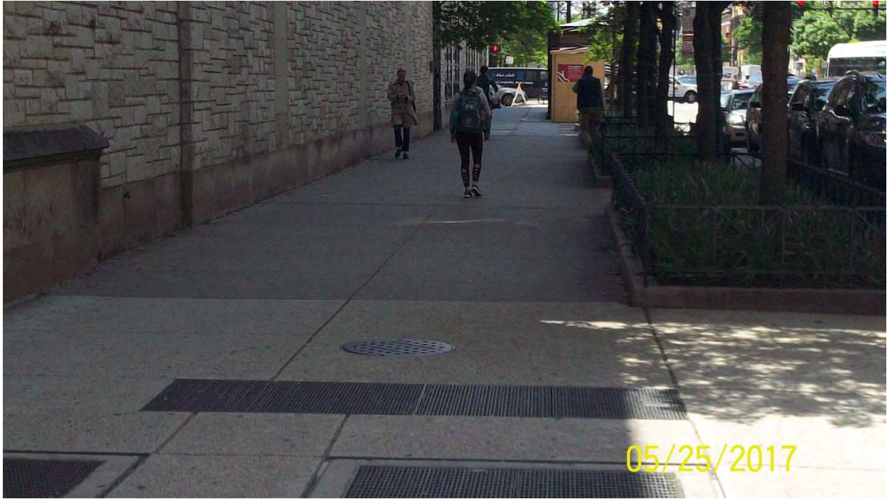
Photo 19: Southwest corner of Chicago Ave. / Wabash Ave. – Looking West
