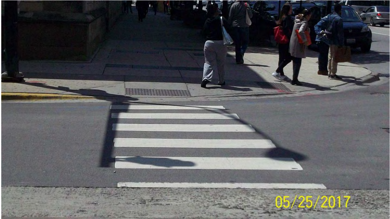
Photo 21: Southeast corner of Chicago Ave. / Wabash Ave. – Looking West
