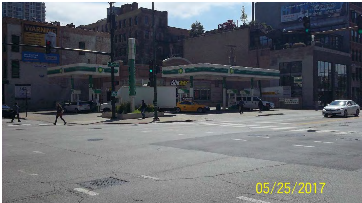
Photo 22: Northeast corner of Chicago Ave. / Wells St. – Looking Southwest
