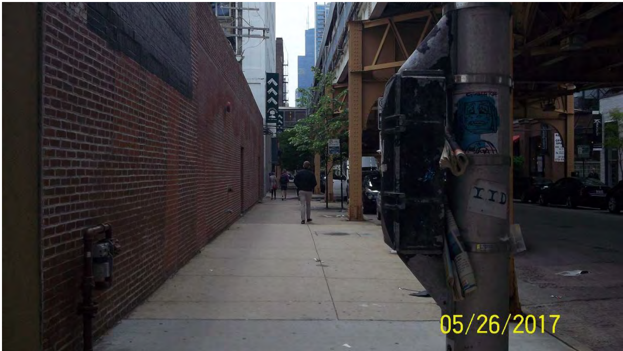
Photo 14: Southeast corner of Chicago Ave. / Franklin St. – Looking South
