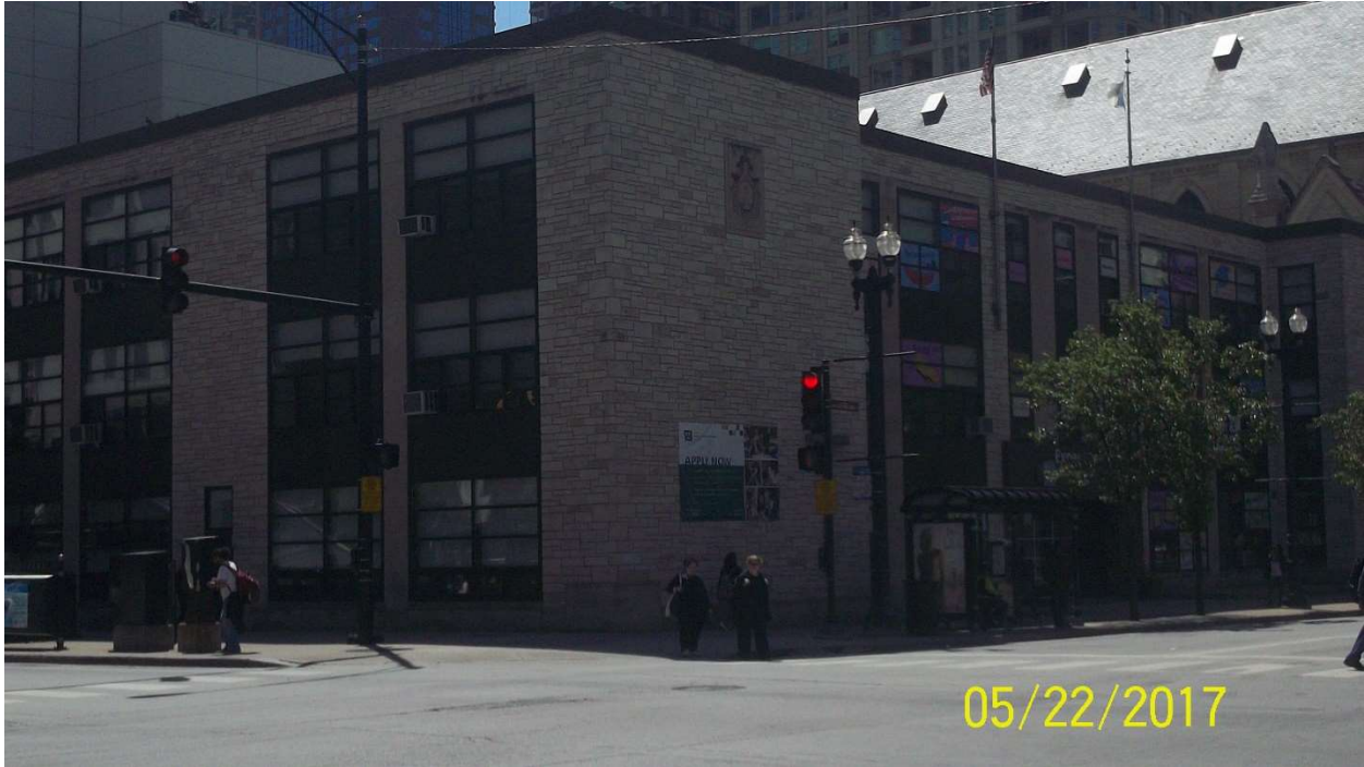
Photo 21: Northwest corner of Chicago Ave. / State St. – Looking Southeast
