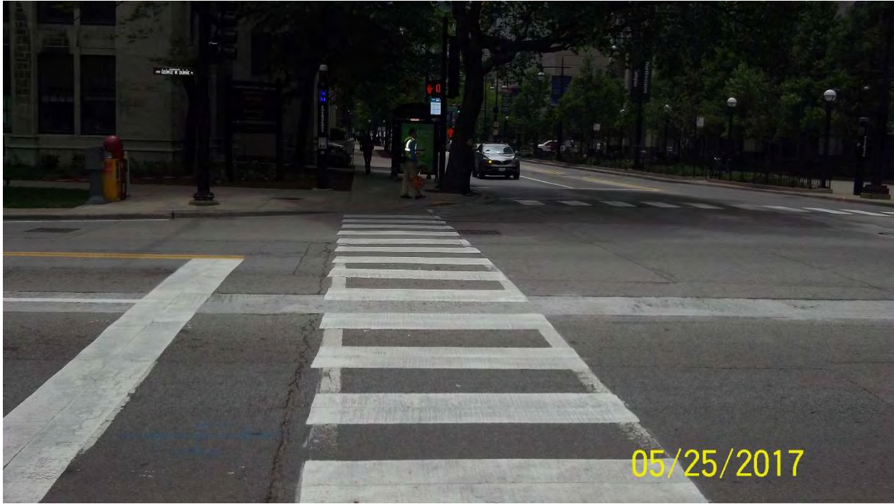
Photo 15: Northeast corner of Chicago Ave. / Fairbanks Ct. – Looking South
