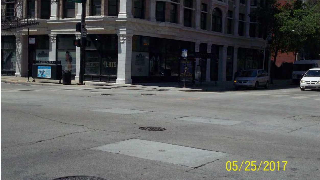
Photo 7: Southeast corner of Chicago Ave. / Clark St. – Looking Northwest
