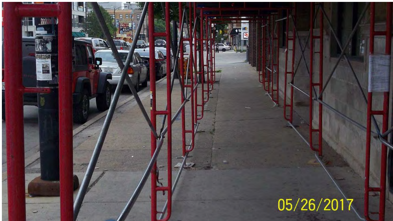
Photo 20: Southeast corner of Chicago Ave. / Western Ave. – Looking North
