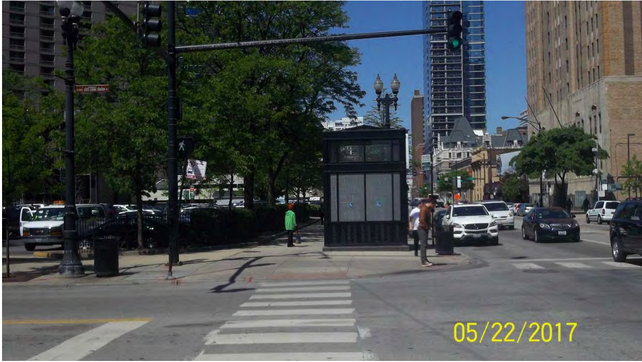
Photo 12: Southeast corner of Chicago Ave. / State St. – Looking West
