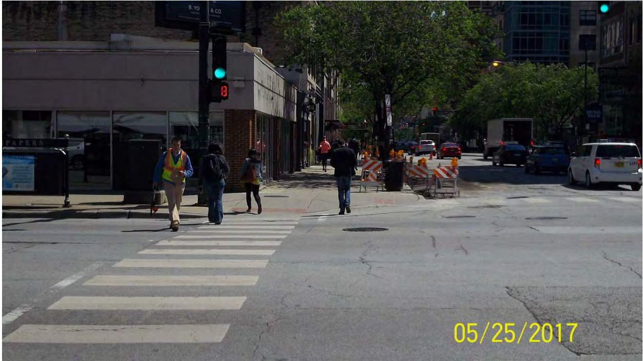
Photo 23: Northeast corner of Chicago Ave. / Clark St. – Looking South
