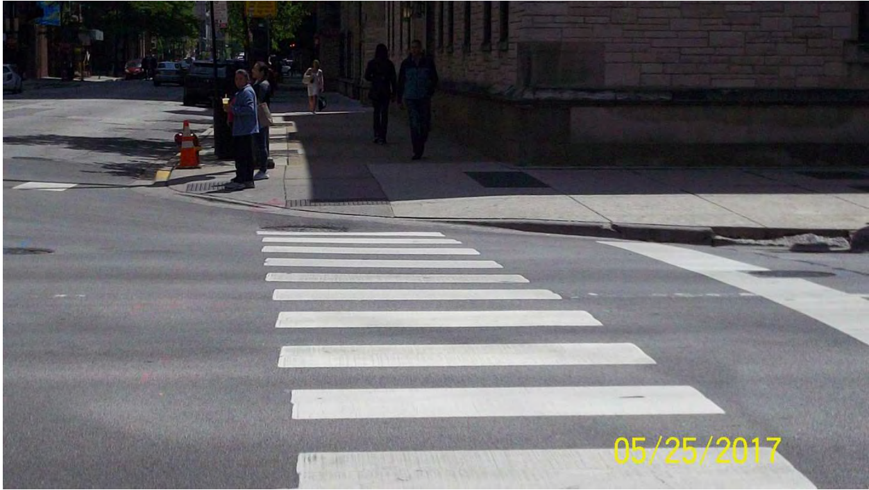
Photo 13: Northwest corner of Chicago Ave. / Wabash Ave. – Looking South
