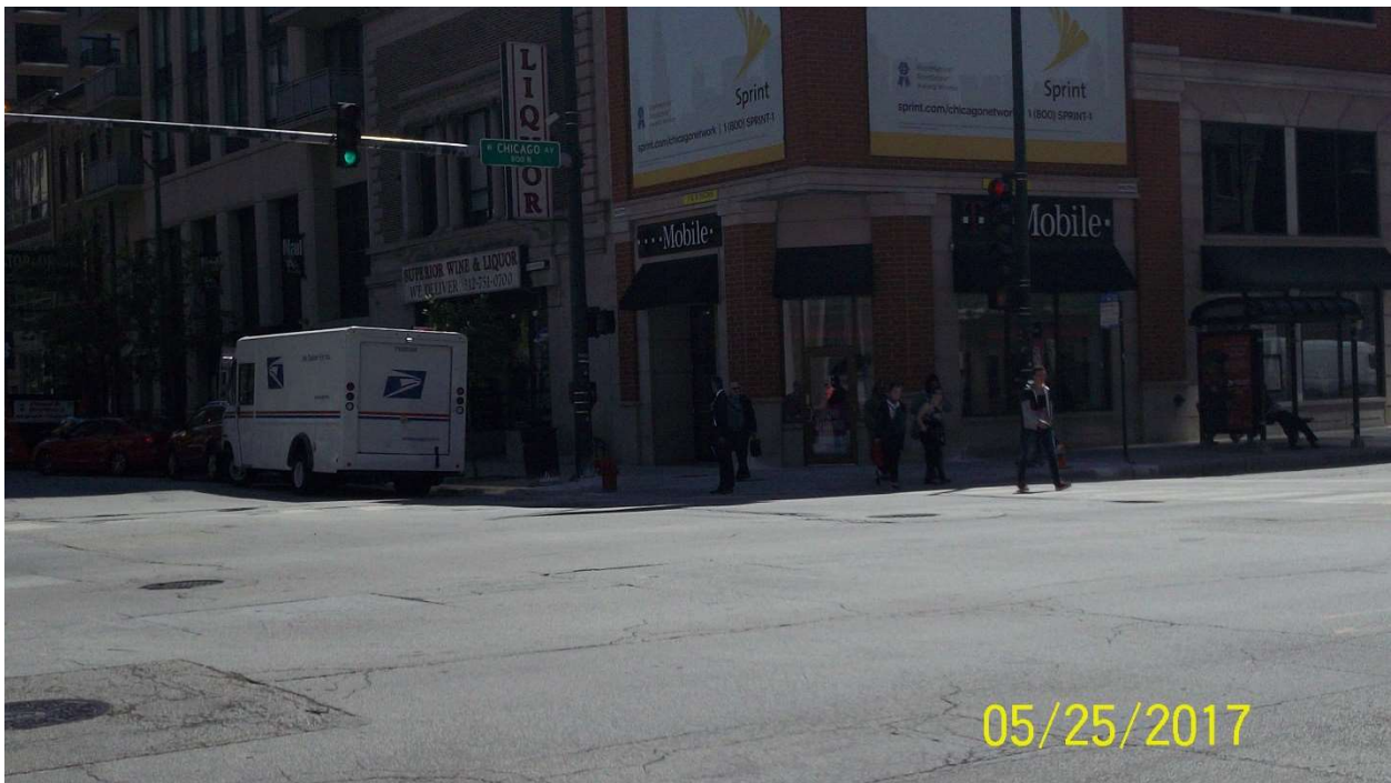
Photo 22: Northeast corner of Chicago Ave. / Clark St. – Looking Southwest
