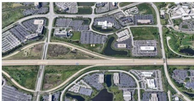
Figure 3 Aerial of typical Naperville-Warrenville Rd development typology
