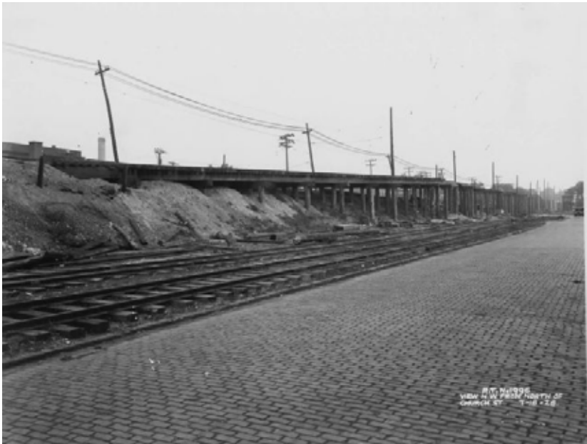
A view to the northwest from Benson just north of Church during the second phase of track elevation in the 1920s. The C&ME's tracks are still at street level in the foreground. (Collection J.J. Sedelmaier Productions, Inc.; M. D. McCarter photo.)
