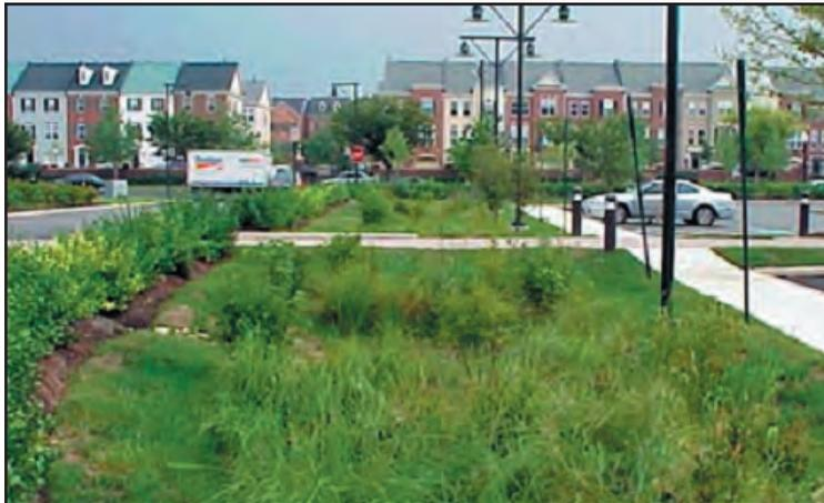
Low maintenance bioswales can be used in open spaces and parking areas to reduce stormwater.
