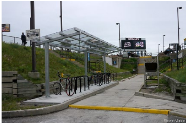
Example: Covered bike parking at the Clybourn Metra Station
