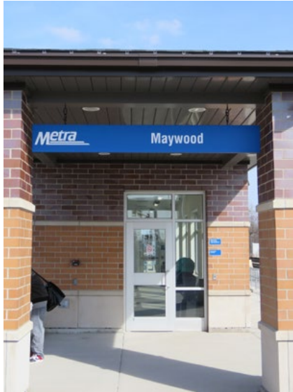
Station signage with lighting
