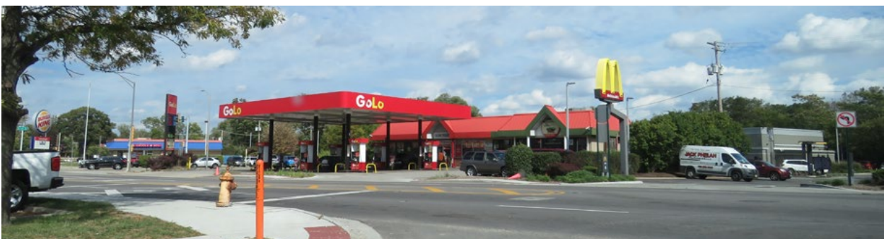
Existing development at the intersection of 1st Avenue and Lake Street prioritize automobiles over pedestrians
