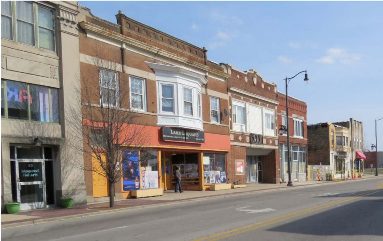
First block of 5th Avenue north of Main Street
