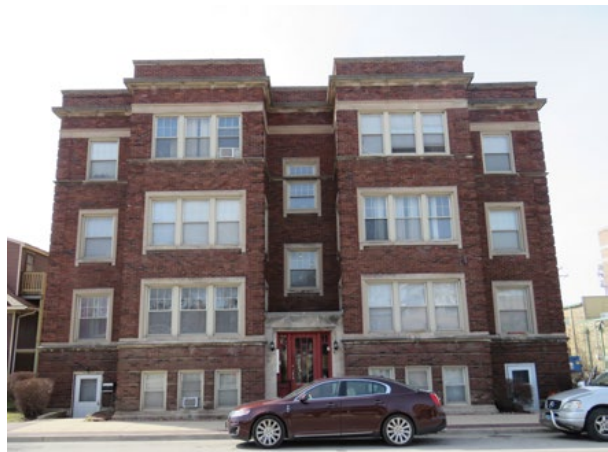
Existing multi-family housing in downtown Maywood
