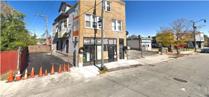
Curb cuts (V1), (V2), and (Y) near 409 W. Lake Street
