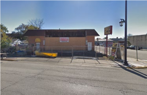
Curb cut (Z) near 320 W. Lake Street
