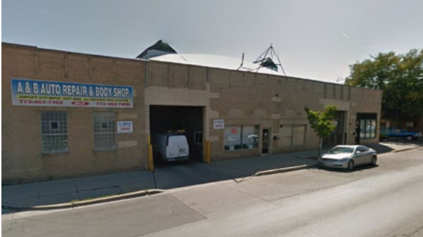
A former auto repair shop converted to an adult and children's fitness studio, with a bar and grill next door in Chicago.
