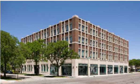
Interfaith Housing Development Corporation, the Oak Park Housing Authority and Catholic Charities developed the vacant former Cadillac-LaSalle Car Dealership in Oak Park into 51 units of supportive rental housing for low-income adults. Sugarbeet Cooperative Grocery Store occupies the first floor commercial space.
