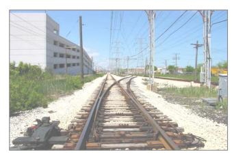
Figure 3-2: Looking north along the west track at the Searle crossover. To the right of center, one of the catenary towers with the supports between the tracks is visible. Above ground utilities in this section of line are evident.
