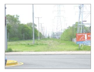
Figure 11-7: Looking north of Dempster, ComEd wood poles run between the station parking lot and the UPRR track and would have to be relocated in order to provide a tangent transit right-of-way of suitable width for a double-track line. This view looks north from the end of the CTA tail track and shows that pole line to the left of center in the view.
