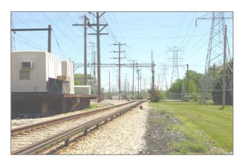
Figure 3-15: The Yellow Line section between Crawford and East Prairie is equipped with both third rail and overhead catenary. The third rail is evident on the outside of the tracks through the site of the former Crawford station platform, which is now used to accommodate a cab signal bungalow.
