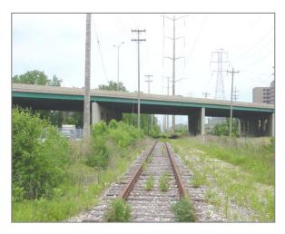
Figure 3-11: Looking north toward the Edens bridge. The former CNS&M catenary tower bases are intact and are located 11 feet west of the track centerline and 24 feet-6 inches to the east, giving a total separation distance of 35 feet-6 inches. These bases would be removed prior to any new line construction.
