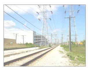
Figure 11-3: This photo, north of Oakton and looking north, shows catenary towers that must be removed for station construction. For the station house and 520-foot platform configuration, there are a total of four catenary towers that would have to be removed. If the station were to extend to Searle, a total of five towers are affected. The Pharmacia parking structure is to the left.
