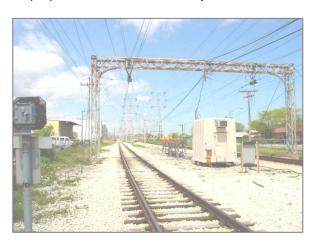
Figure 11-6: An example of a betweentracks signal relay house installation is on the north side of Oakton. This example is a much smaller relay house footprint, compared to the 550 square foot requirement referenced in the text.
