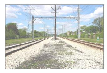
Figure 3-1: Looking west from Crawford Avenue. The catenary towers with the vertical supports outside of the tracks are prominent. Also evident are the various aboveground utilities on the ROW.
