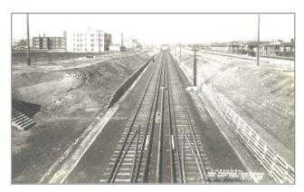
Figure 9-1: This construction-era photograph of the existing Yellow Line open cut through Evanston shows the angle of the side slopes.
