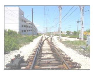
Figure 11-4: Looking north from Oakton, the emergency crossover and the cantilever style of catenary towers are pictured. Wood poles adjacent to the right-of-way may require relocation or rerouting, depending on the length of the station at Oakton Street. Pharmacia's parking structure is to the left.
