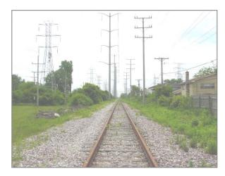
Figure 3-10: The 33-foot separation distance between the wood pole line and the first of the high-tension lines is sufficient for a double-track rail line, so long as this does not include station platforms.
