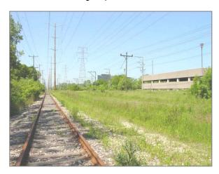
Figure 3-12: A former CNS&M siding was located to the east of the main track at one time. At the time of inspection, wood poles with the span arms (once used to hang the trolley wire over the siding) were still in evidence.
