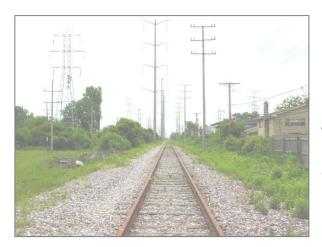
Figure 11-8: On the south side of Golf Road, the high-tension pole line is 17 feet-6 inches to the west of the UPRR track centerline. The pole line runs approximately down the middle of this photo. The wood pole line to the west of the UPRR is about 13 feet-6 inches removed from the track center. This gives an overall width of 31 feet between the poles. This view looks south from the Golf Road grade crossing.
