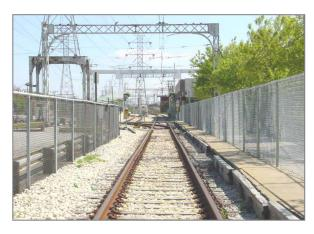
Figure 3-3: Looking south at the Dempster tail track. Old and new catenary towers are evident. The square tower base to the left of the view once had a CRT terminal track passing under it, hence the unusual design.
