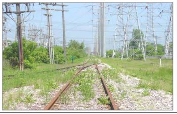
Figure 3-9: In the vicinity of the north end of the siding. Double tracking in this area would require relocation of many of these towers and poles.
