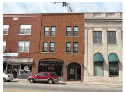
Complementary building forms and retail streetscape character.
