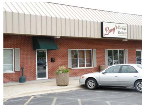
Unattractive/ disproportionate retail storefront facade character.
