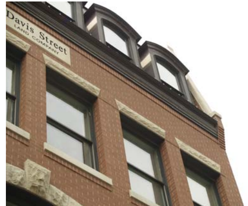
Well-articulated and proportional upper floor fenestration.
