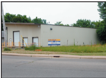
Vacant warehouse building
