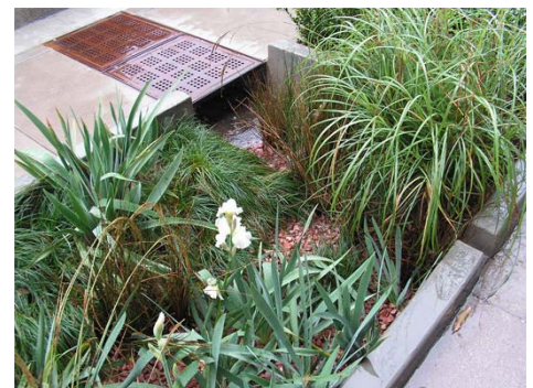
Bioswales and best practices in stormwater management shall be considered in all new site development.
