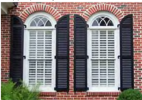
Appropriately Scaled Shutters: Permitted
