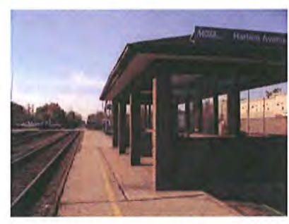
The warming shelter on the outbound track.
