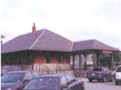
The Berwyn station building, located on the inbound track, is a historic landmark building from 1890.
