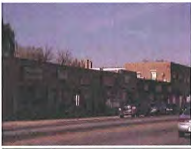
Typical one & two story brick commercial buildings.
