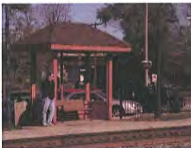
The warming shelter on the outbound track at the LaVergne station.
