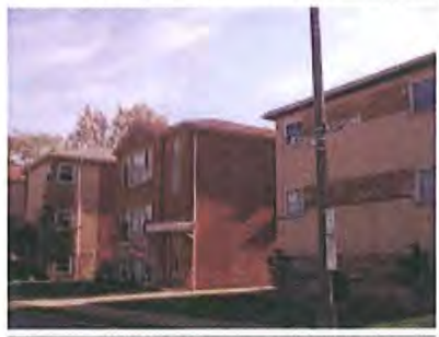
Three story brick multifamily buildings line both Windsor and Stanley Avenues close to Harlem Avenue.
