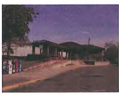
The station building is located immediately adjacent to the Windsor Street cartway, too close to the travel path of vehicles.
