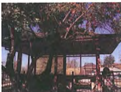
The LaVergne station inbound track warming shelter.
