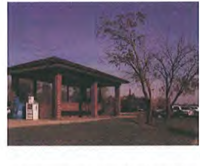
The warming shelter on the inbound track.
