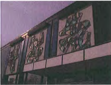
The Berwyn Community Bank building on Oak Park Avenue had the above art piece commissioned, and is now considered a local landmark.
