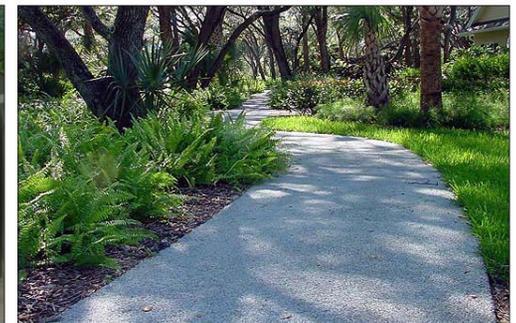
Although still a hard surface, pervious concrete allows water to flow through the material more freely, meeting EPA stormwater management standards.
