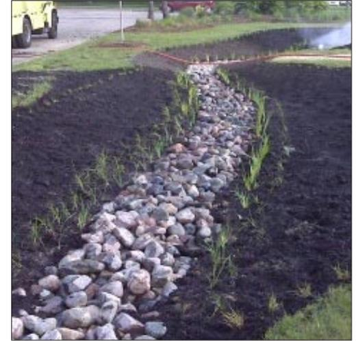
*A rain garden is a vegetated depression that helps reduce stormwater runoff by filtering rain back into the ground to maintain the natural cycle of water. A rain garden can be placed near buildings, in parkways, and in and around parking areas.*
