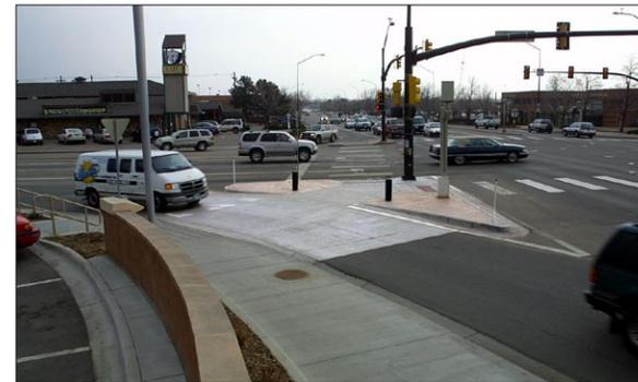
Figure 1.14: Photo showing raised channelize right-turn lane with pedestrian refuge area
