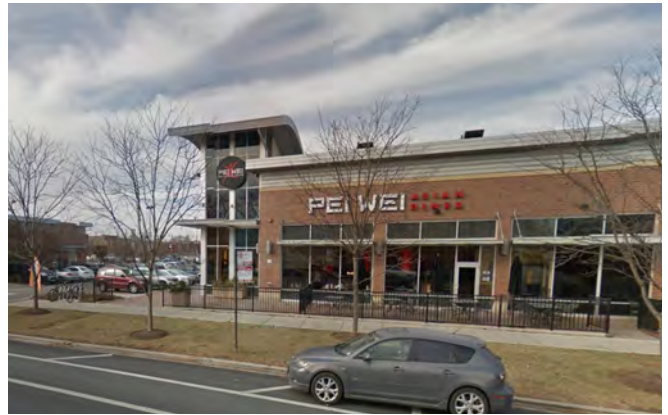
New Construction, Single Story, Commercial Center Storefront Building
