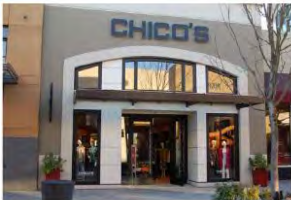
Commercial Grade Doors & Windows on Commercial Buildings.
