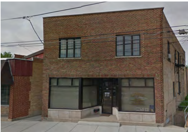
Existing Historic Storefront Building
