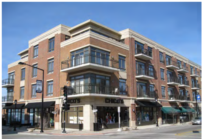
New Construction, Mid-Scale Storefront Building
