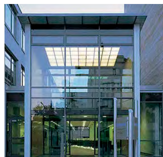
Glass Curtain Wall
