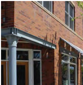
Brick with Metal Details
