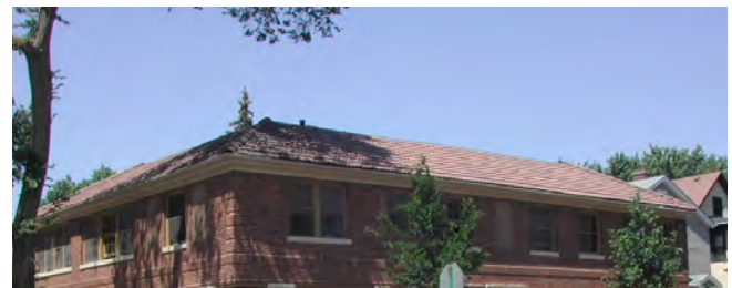
Roof Materials: Ceramic Tile
