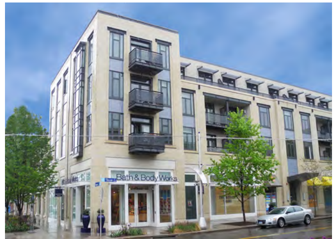
New Construction, Mid-Scale Storefront Building
