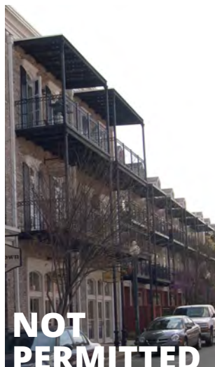
Balconies: Covers More than 40 Percent of Facade
