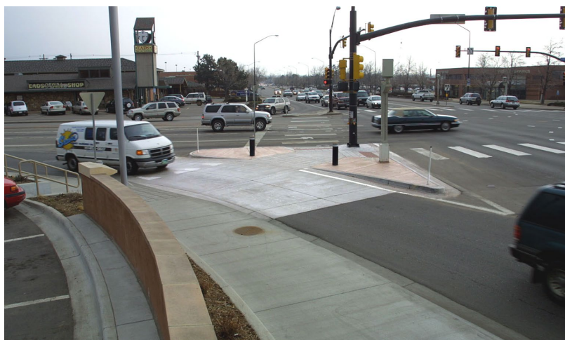
Figure 23 – Example of a ‘pork chop’ refuge island. Note the yield sign and the protective bollards. Source: Dan Burden, CMAP Complete Streets Toolkit
