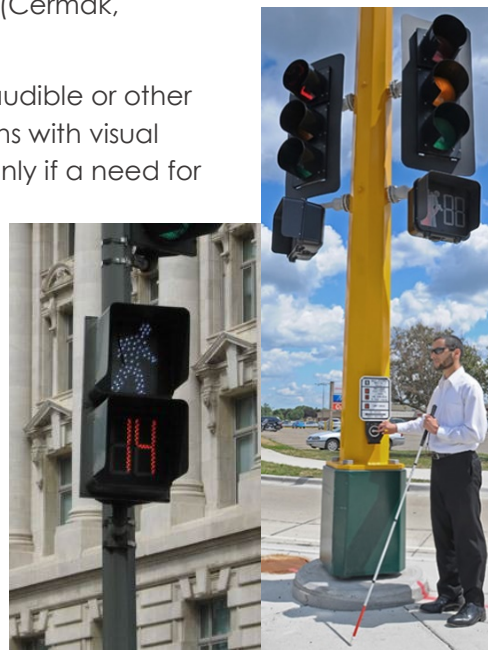
Figure 18 - Countdown Signals and Accessible Pedestrian Signals. Source: IDOT Bicycle and Pedestrian Toolbox and MNDOT
