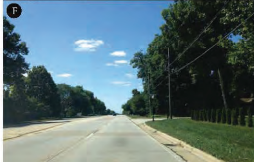
Pedestrian walks are lacking along segments the corridor
