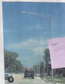
Existing Roadway Lighting
