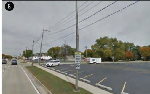
Perimeter and internal parking lot lacks landscape and screening
