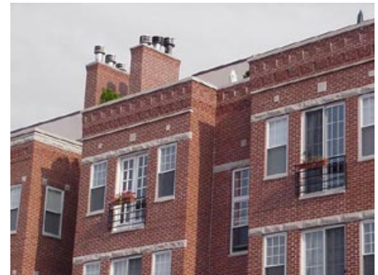
Stone, simulated stone, and precast concrete are among the recommended accent materials.
