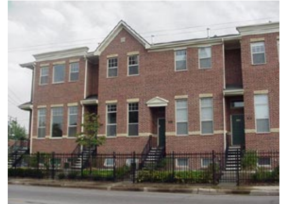
This multi-family building features a parapet wall and flat roof profile, a series of projecting bays that breaks up the bulk of the building, and prominent, inset entrances. Recommended landscape elements include the metal fence and buffer of low evergreen shrubs.
