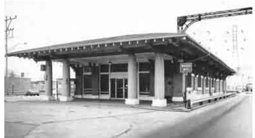
Dempster Street Station in Original Location, circa 1990
