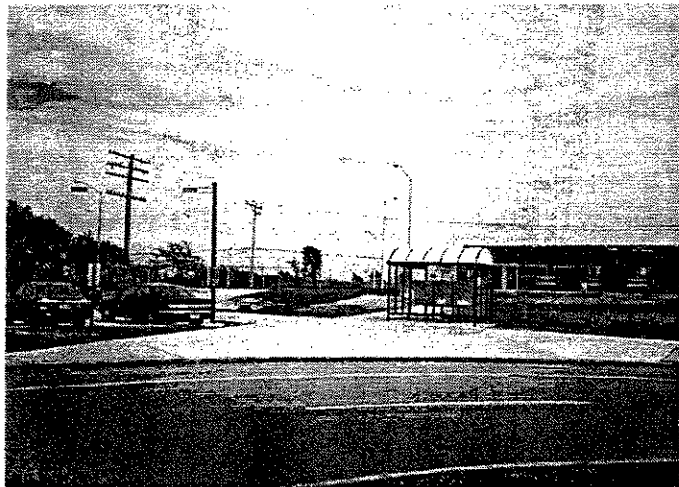
Figure 21: The temporary ramp and walkway near the Kiss n’ Ride lane on the north side of the tracks, with the 80th Avenue station facility visible on the right and the north parking lot visible on the left.
