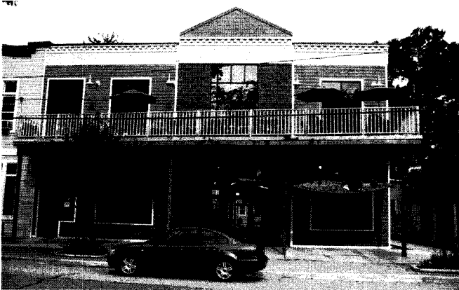
Primary Materials: Painted Wood
