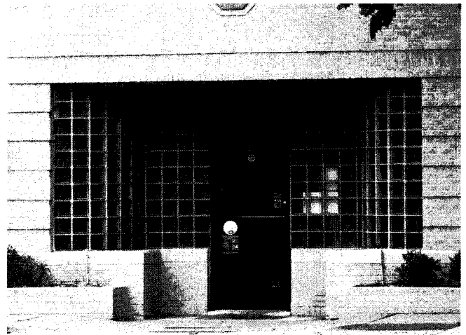
Prohibited: Glass block windows on front facade.
