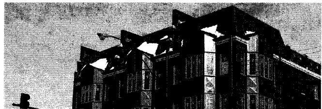
Roof Materials: Metal
