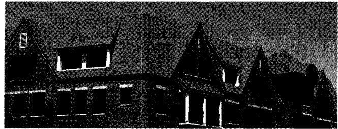
Roof Materials: Asphalt Composite Shingles
