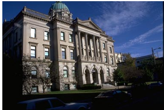
Adjectives: wonderful; historic Characteristics: 4-stories; limestone; set back from street; well-kept landscaping
