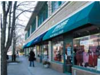
Buildings east of the tracks generally appear to be in good condition.
