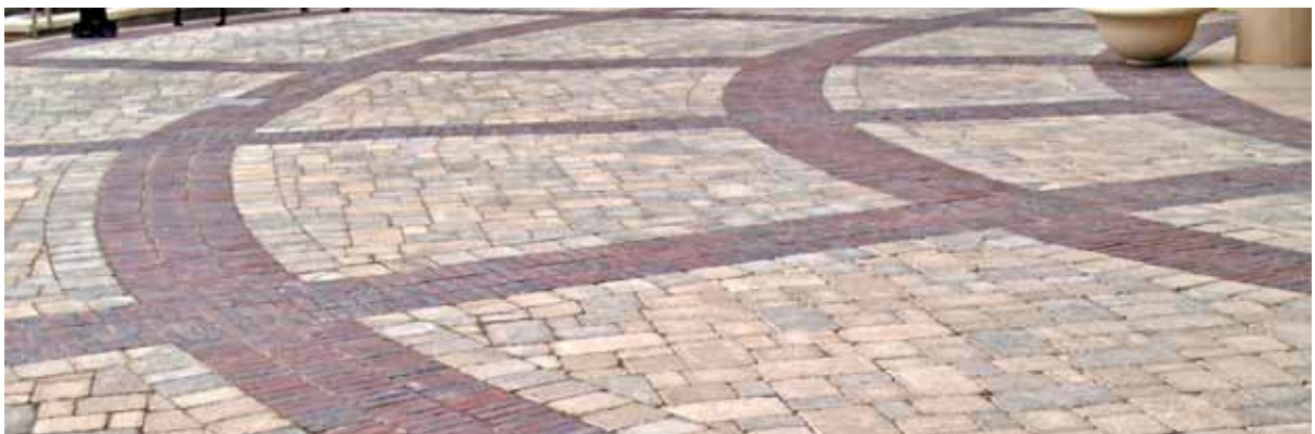
High quality paving materials like brick, clay pavers, stone or stamped concrete should be used in designs for hardscape.
