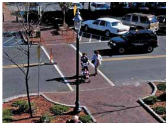
All pedestrian crosswalks should be a minimum of ten feet wide and clearly delineated with striping and/or paving.
