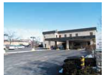
Drive-thru at Premier Bank
