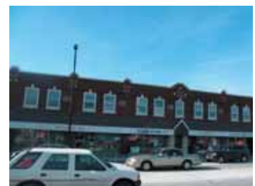
Commercial along Green Bay Road
