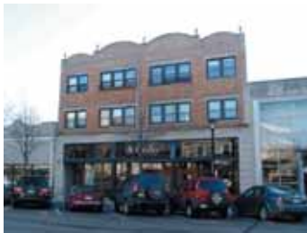
Example of commercial/mixed-use building east of the tracks
