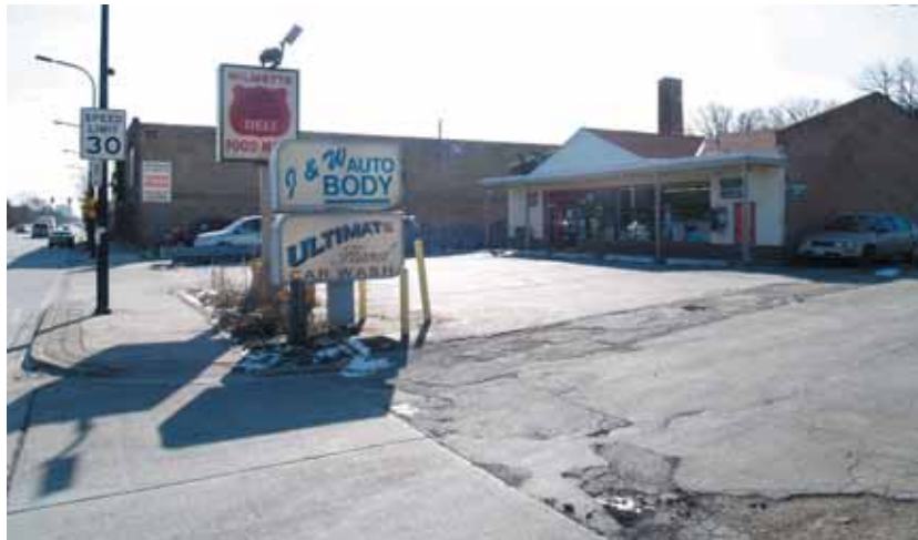
The block south of Wilmette Avenue has multiple curb cuts and excessive parking.
