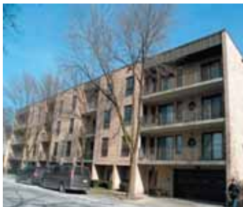
Multi-family residential building on 12th Street
