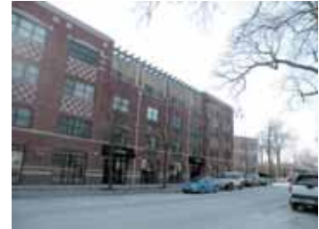
The Verona condominium building
