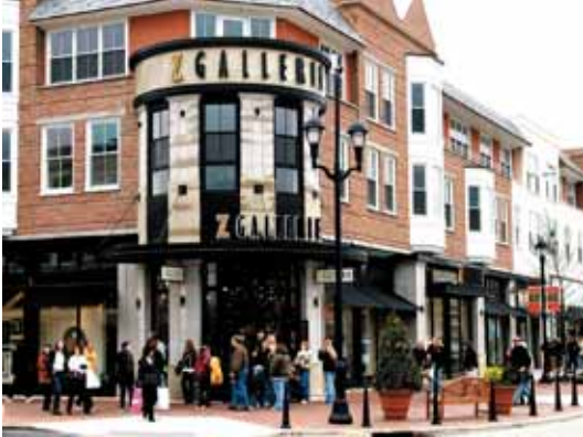
New developments should hold the corners of intersections to enhance the sense of enclosure and pedestrian-orientation.
