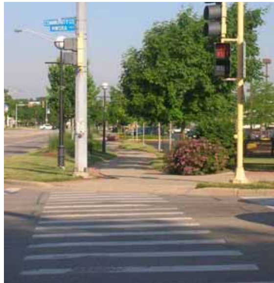
Pedestrian crossing with continental style pavement marking.
