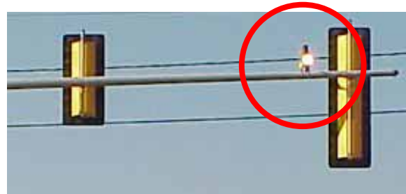
Transit signal priority beacon (top) and activated by a vehicle (bottom). Source: Village of Mount Prospect.
