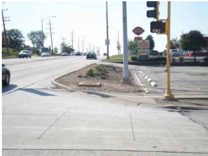
Existing roadside conditions along La Grange Road at 144 th Street.
