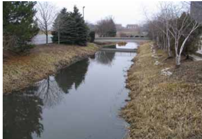
Open stormwater drainage integrated with landscaping near in the South-Center section near 156 th Street
