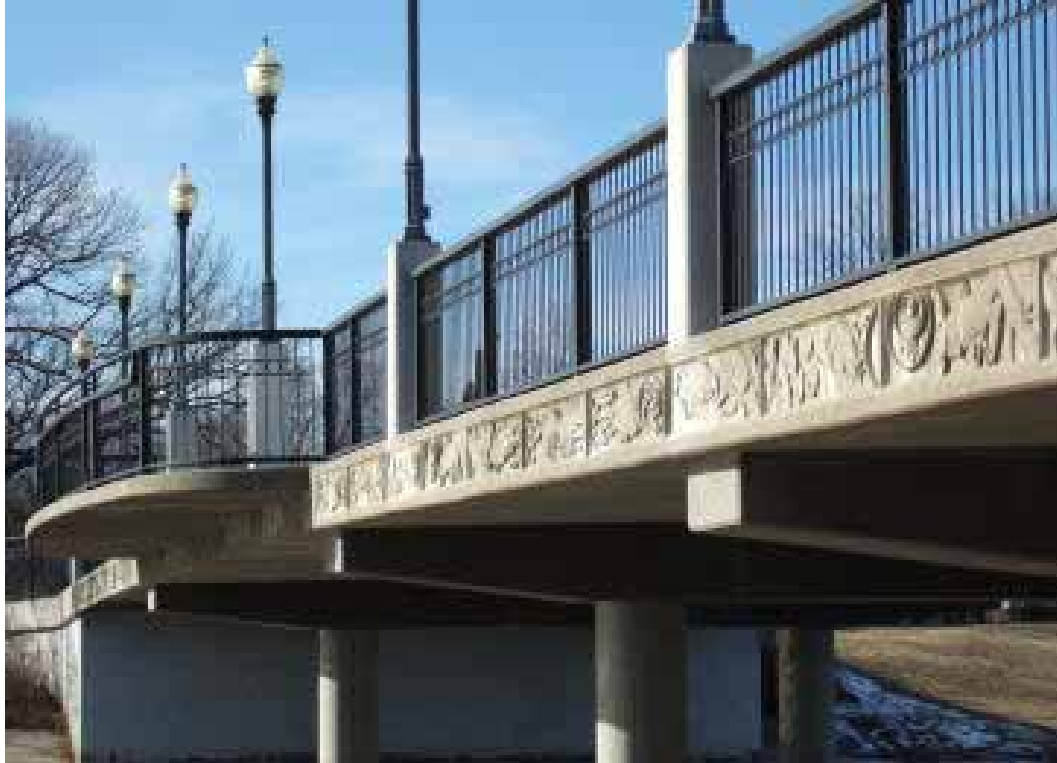
Example of carved façade bridge treatment. Source: Wichita State University. 2003.
