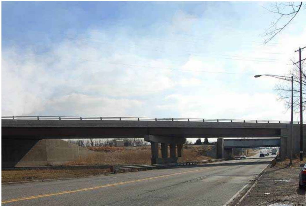
Existing Southwest Highway Bridge
