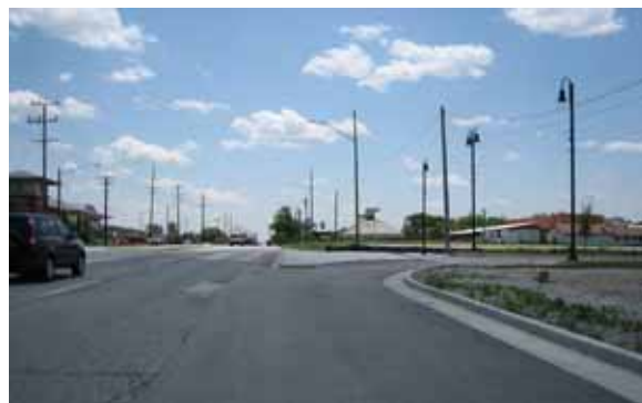
Overhead wires along La Grange Road at 142 nd Place.
