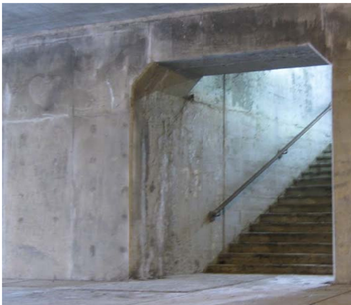
Figure 5-12: Metra Electric District Main Line 95th Street Station Entrance
