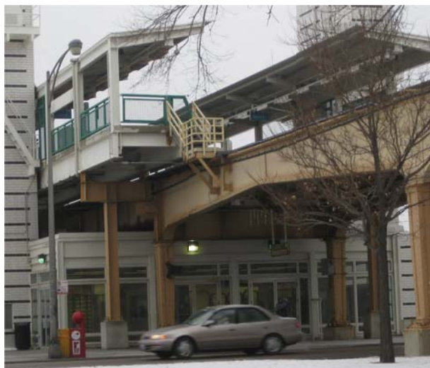
Figure 5-6: CTA Green Line Garfield Station Entrance
