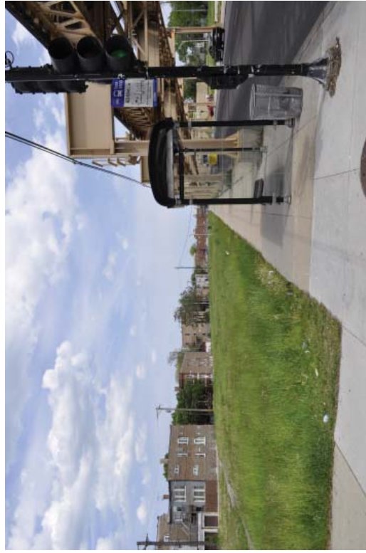
PEDESTRIAN WALKS View looking East on 63rd Street. Bus Shelters and signals interrupt the pedestrian flow. The signals are difficult to see.
