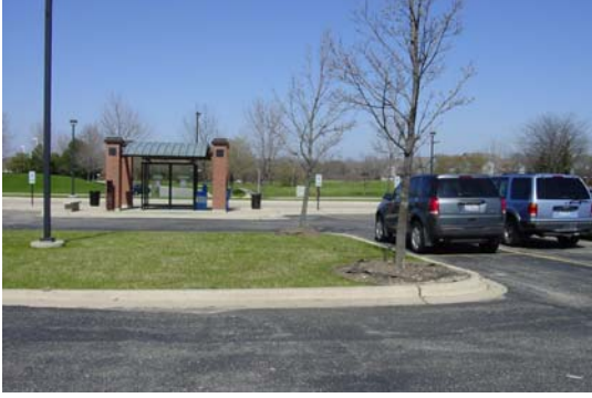
The Pace park-and-ride facility in Burr Ridge, located east of the County Line Square shopping center off of County Line Road south of I-55, provides a dedicated off-street access lane for buses, separate driveway access to a parking lot for commuters, and a shelter for waiting passengers. Businesses are located nearby, but are not integrated with the Pace facility.
