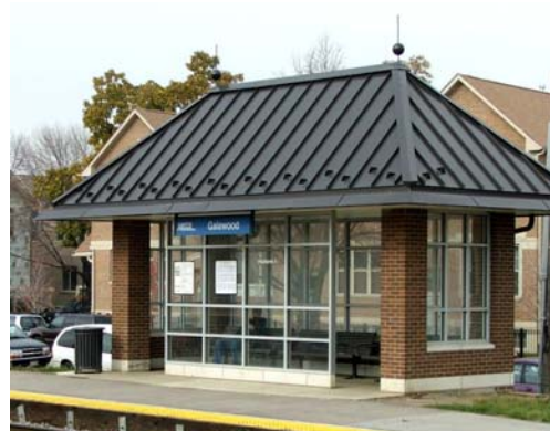
This open but heated shelter at the Galewood Metra Station is a good example of the type of platform shelter that could be constructed at the Justice Metra Station.
