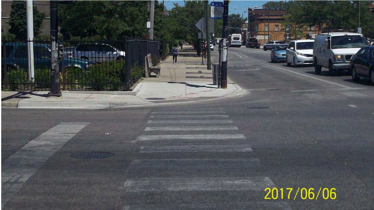
Photo 11: Southwest corner of 79 th St. / Halsted St. – Looking North
