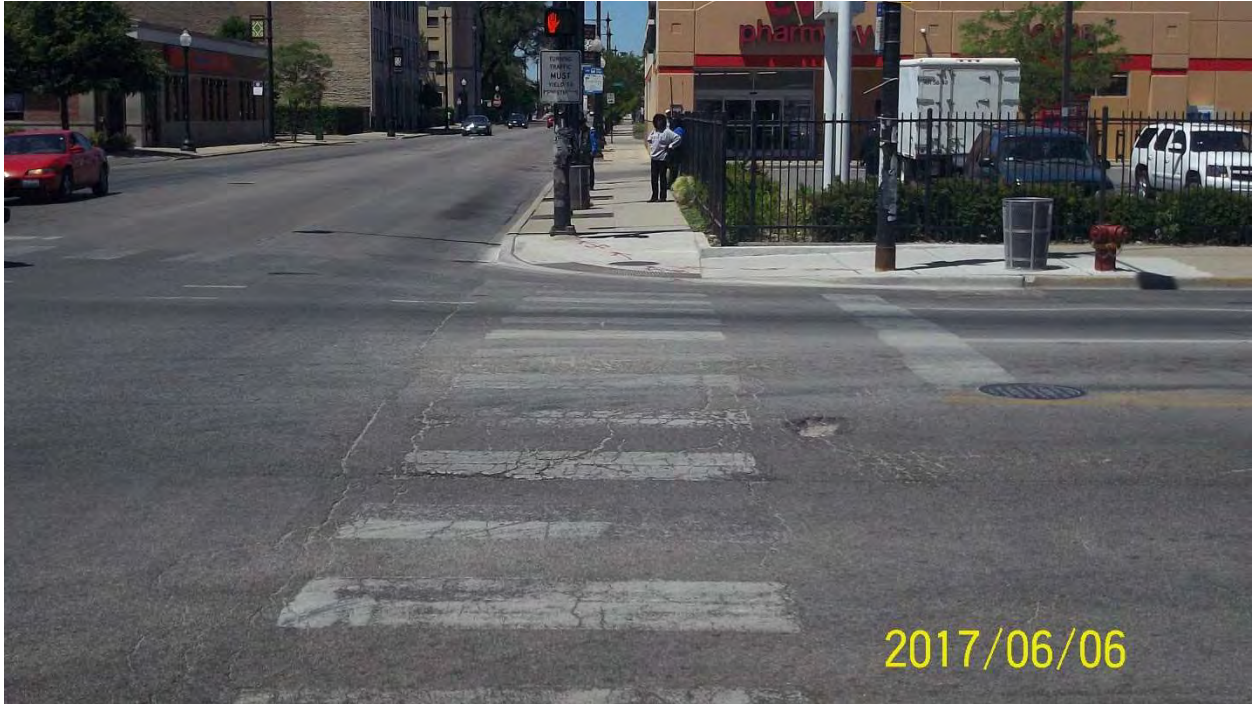
Photo 21: Northeast corner of 79 th St. / Halsted St. – Looking West
