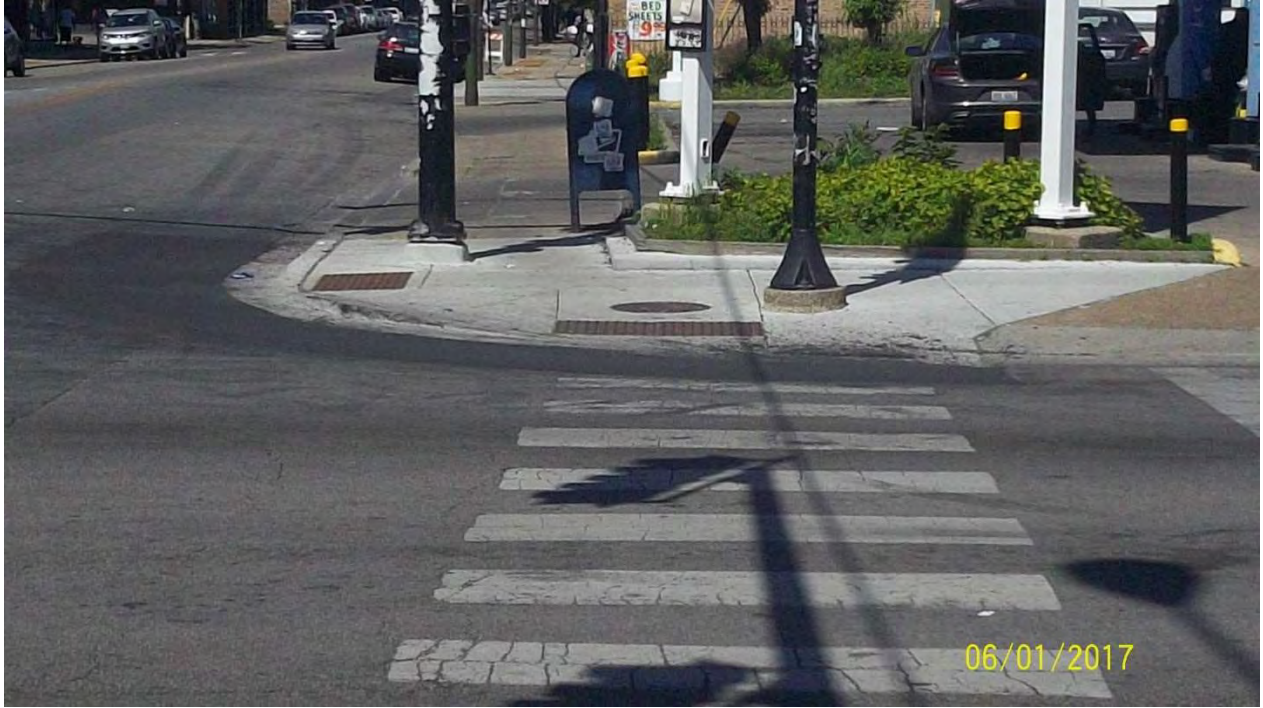
Photo 13: Northeast corner of 79 th St. / Martin Luther King Drive – Looking West
