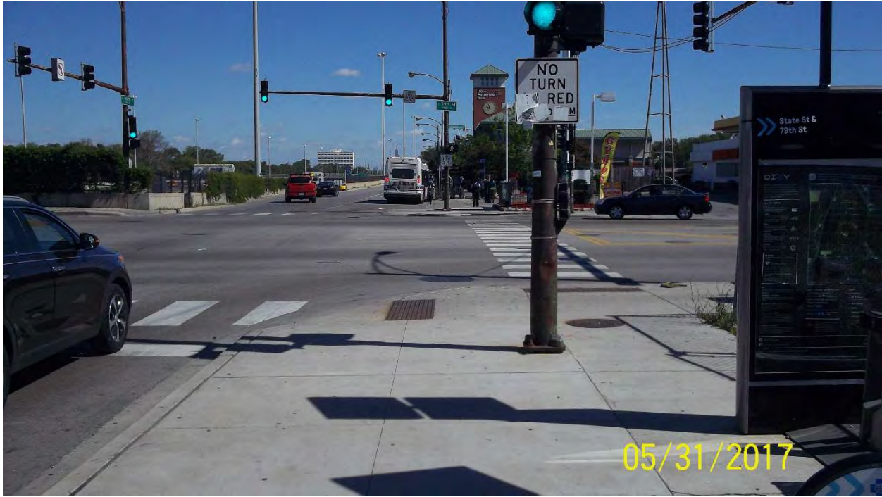
Photo 11: Southeast corner of 79 th St. / State St. – Looking North
