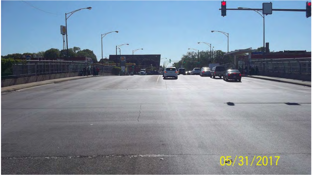
Photo 1: 79 th St. – Looking East
