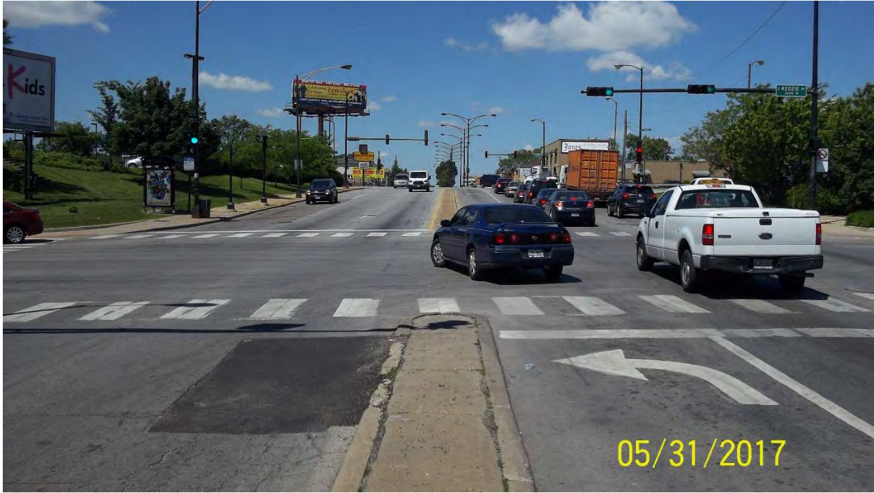
Photo 1: 79 th St. – Looking West
