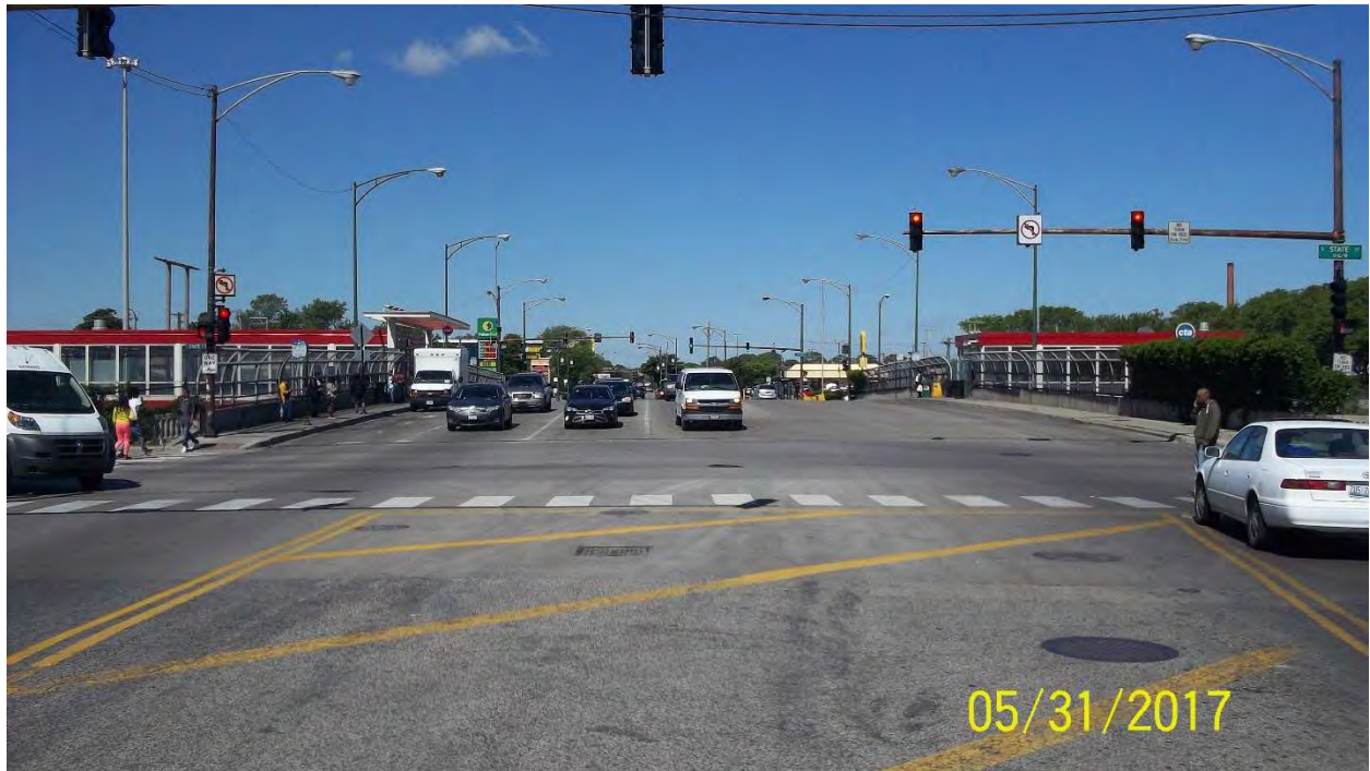
Photo 3: 79 th St. – Looking West
