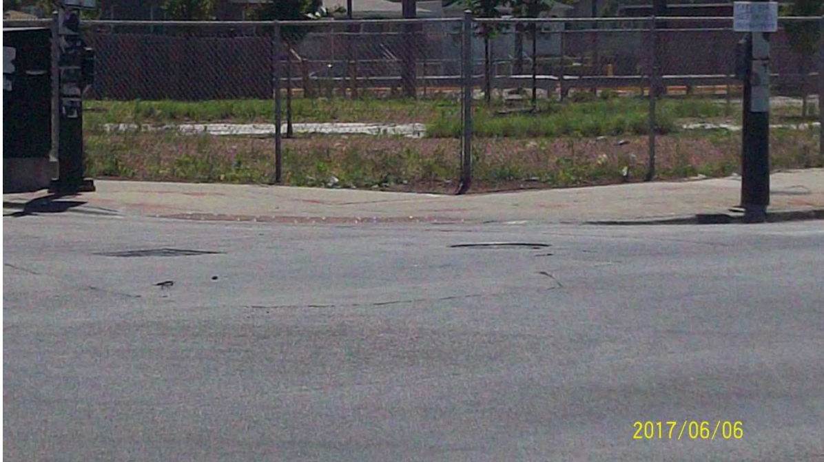
Photo 7: Northwest corner of 79 th St. / Halsted St. – Looking Southeast
