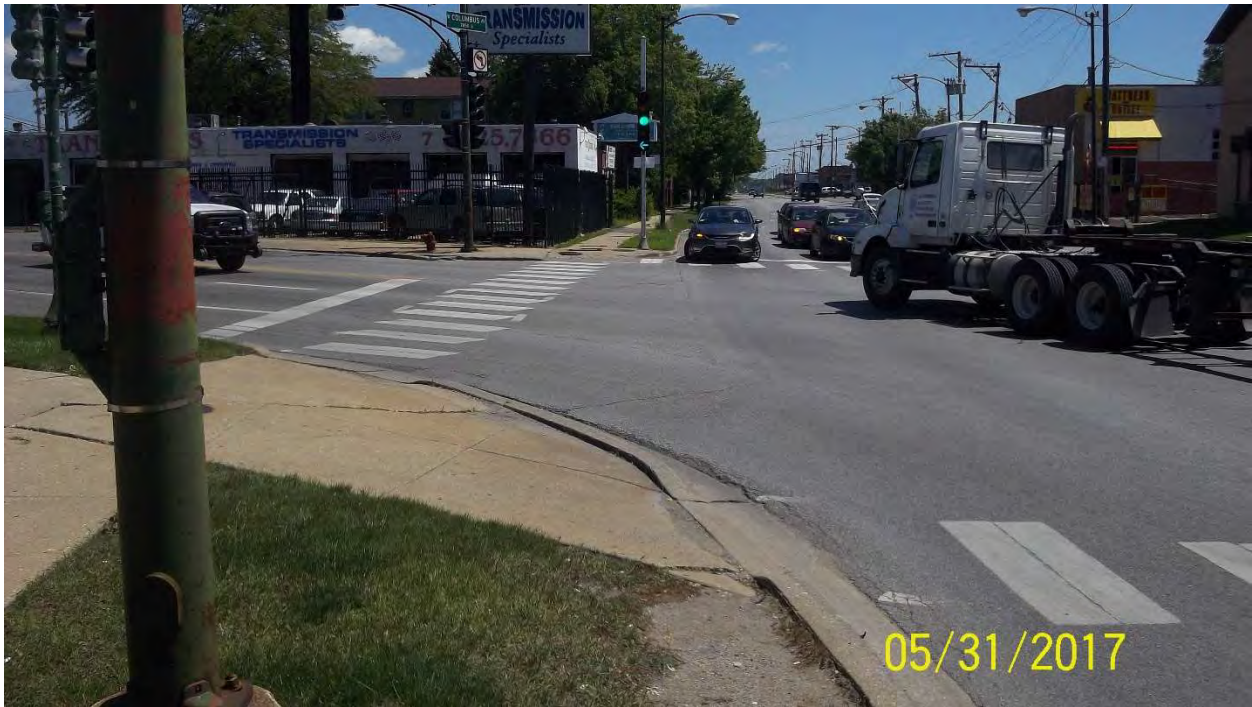
Photo 51: Northwest corner of Kedzie Ave. / Columbus Ave. – Looking East
