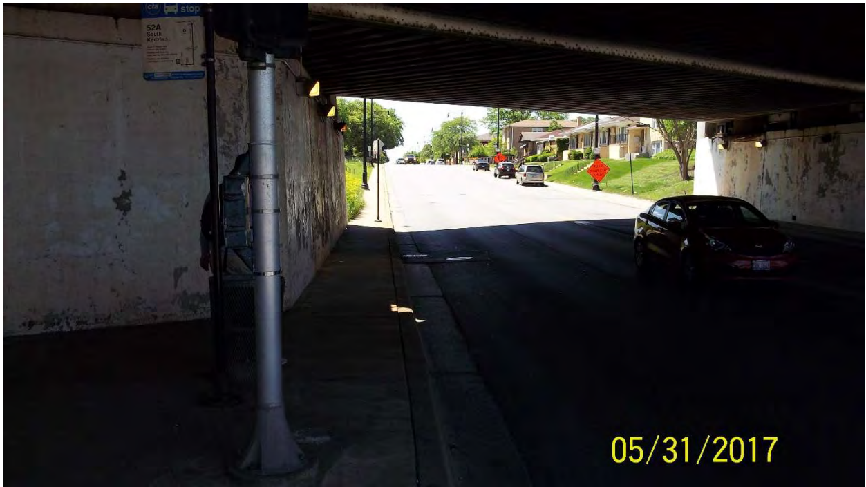
Photo 28: Southeast corner of 79 th St. / Kedzie Ave. – Looking South
