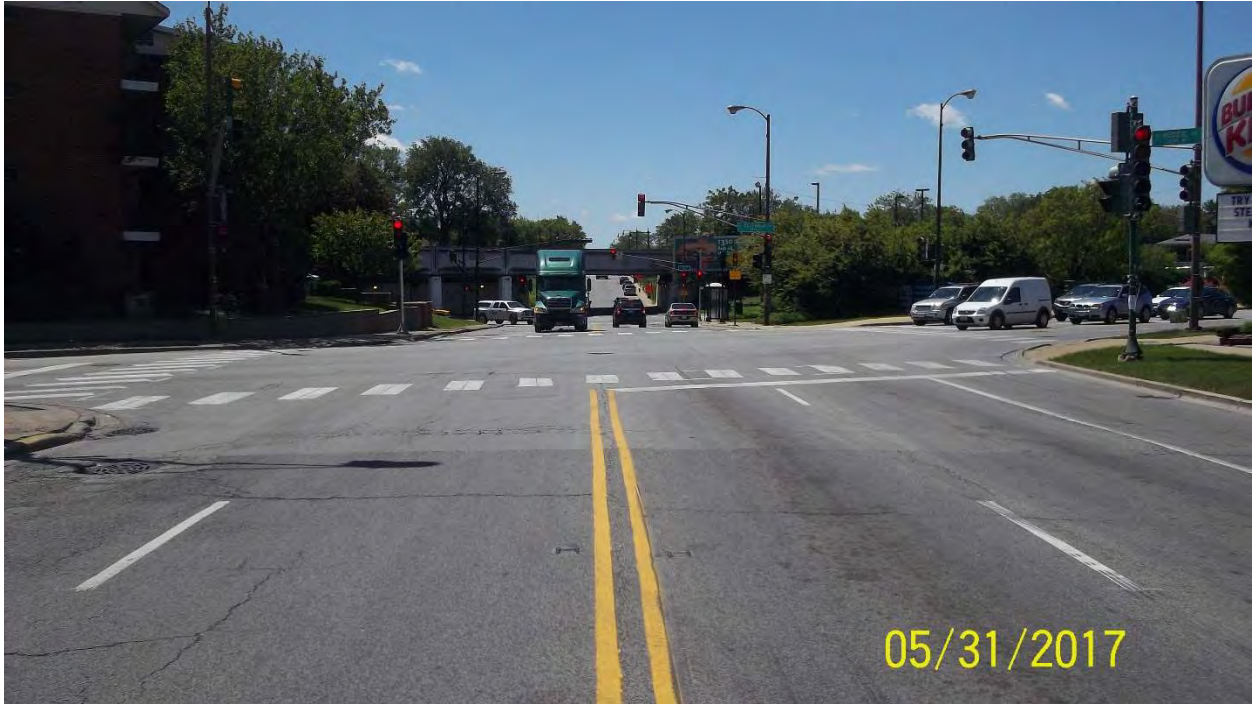
Photo 7: Kedzie Ave. North of Columbus Ave. – Looking South
