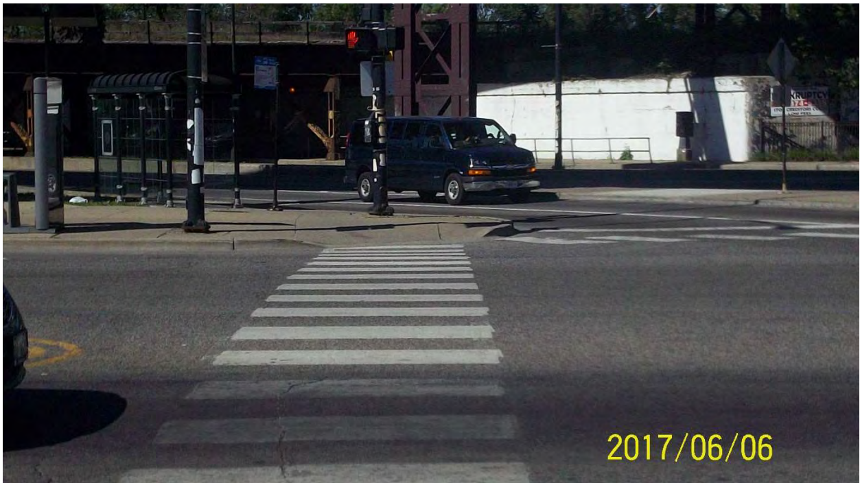
Photo 14: Southeast corner of 79 th St. / South Chicago Ave. – Looking Southwest
