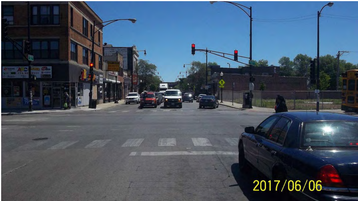
Photo 2: 79 th St. – Looking East
