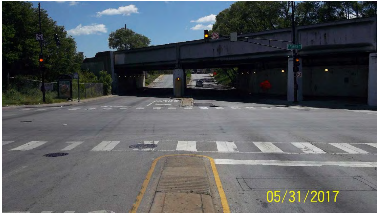
Photo 3: 79 th St. – Looking East
