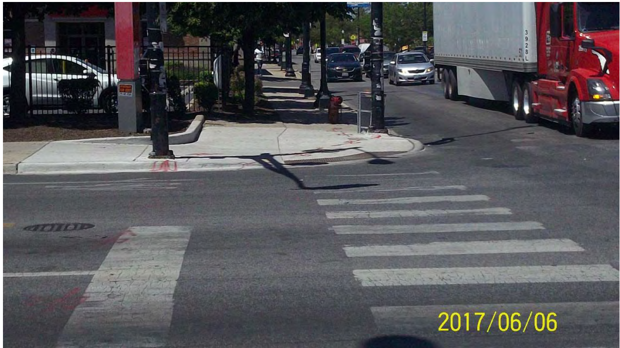
Photo 18: Southeast corner of 79 th St. / Halsted St. – Looking West
