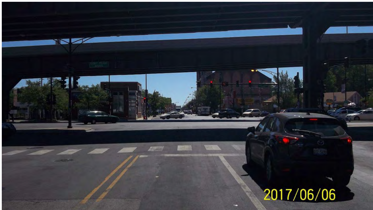
Photo 6: 79 th St. – Looking East
