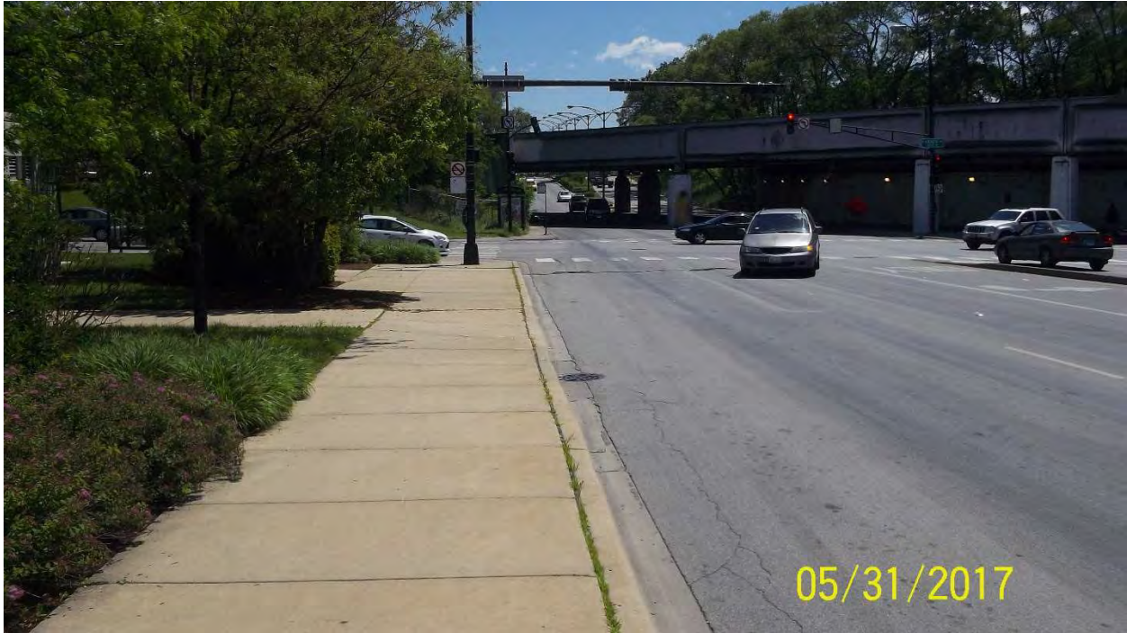
Photo 57: Northeast corner of 79 th St. / Columbus Ave. – Looking East
