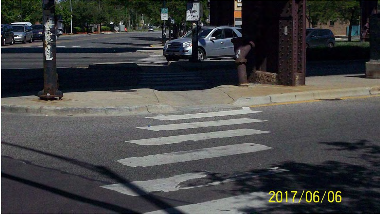
Photo 39: Northeast corner of 79 th St. / South Chicago Ave. – Looking Northwest
