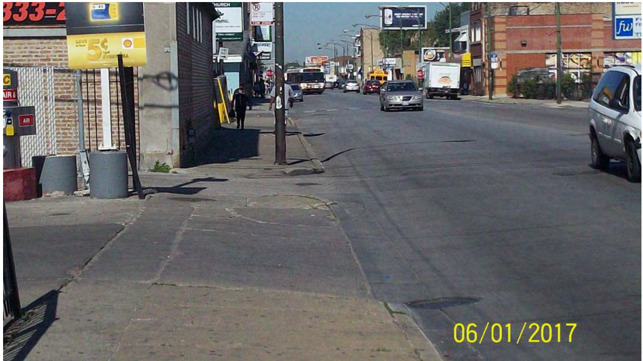
Photo 9: Southwest corner of 79 th St. / Ashland Ave. – Looking West
