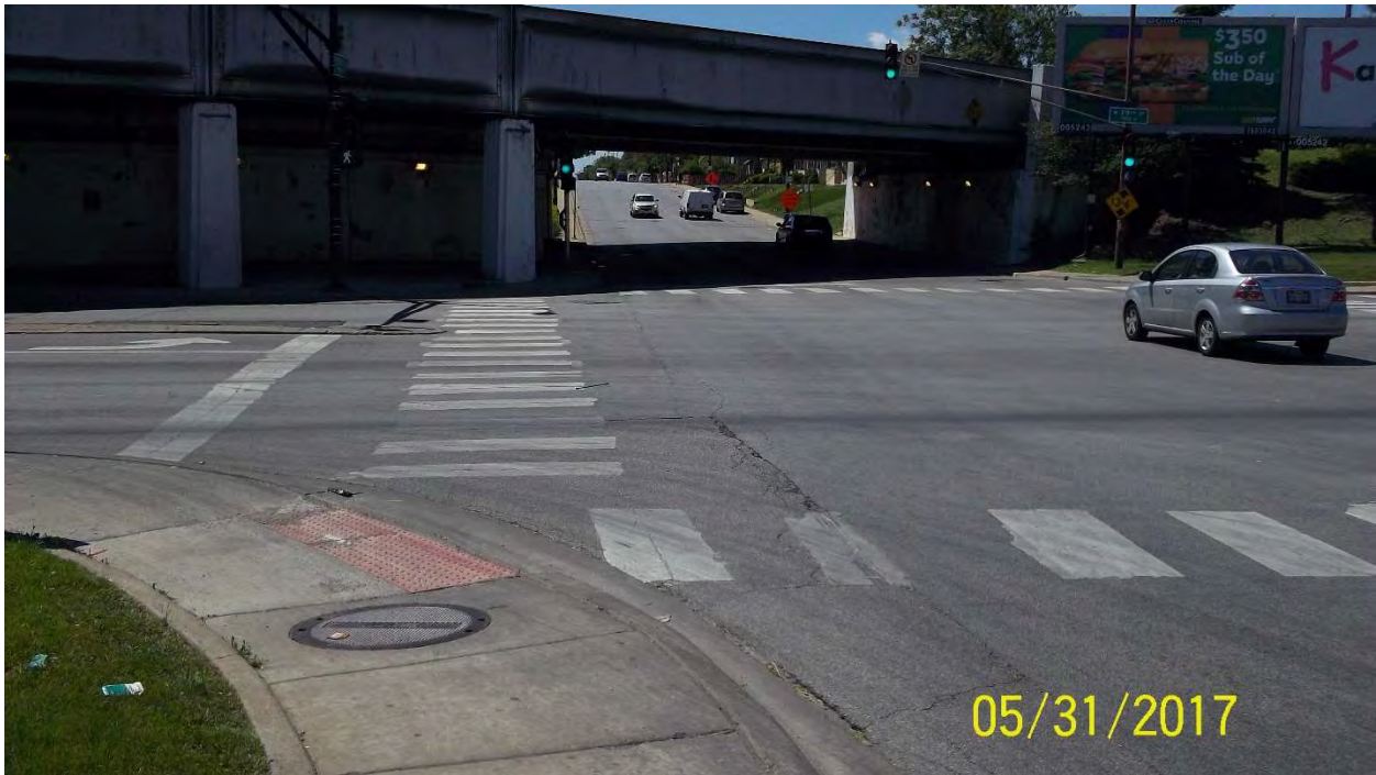
Photo 16: Northeast corner of 79 th St. / Kedzie Ave. – Looking South
