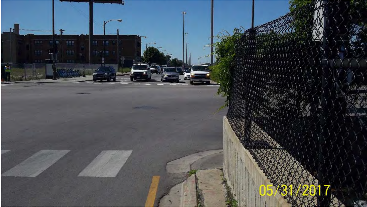
Photo 21: Northwest corner of 79 th St. / State St. – Looking South
