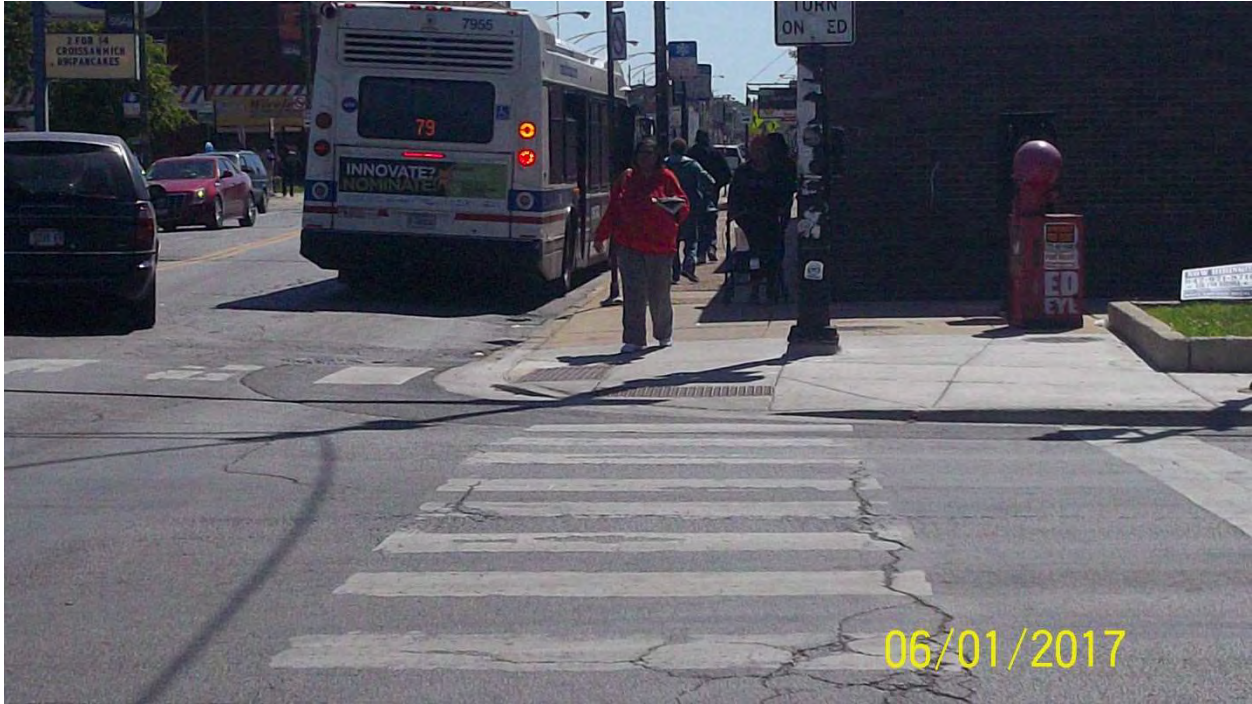
Photo 23: Southwest corner of 79 th St. / Martin Luther King Drive – Looking East
