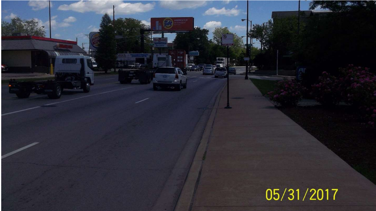
Photo 53: Northeast corner of 79 th St. / Columbus Ave. – Looking Northeast
