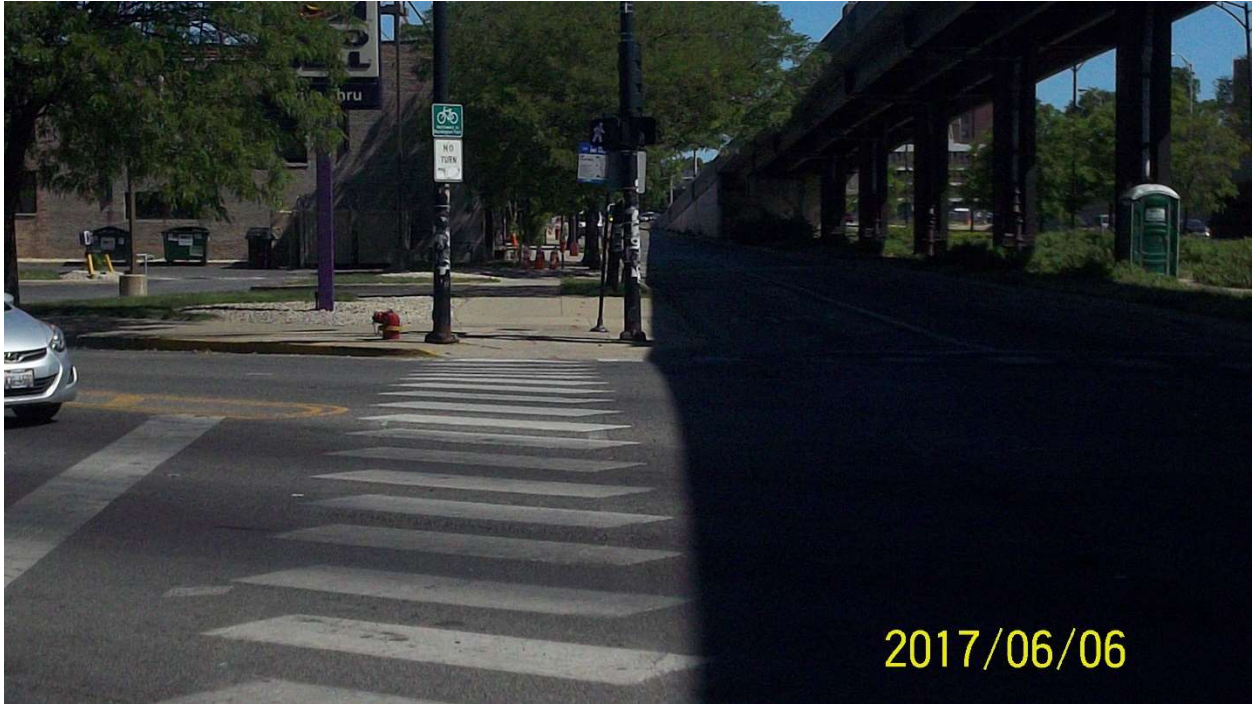
Photo 29: Northwest corner of Stony Island / South Chicago Ave. / 79 th St. – Looking North
