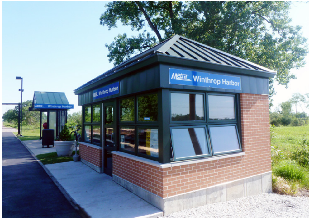
Winthrop Harbor Metra station
