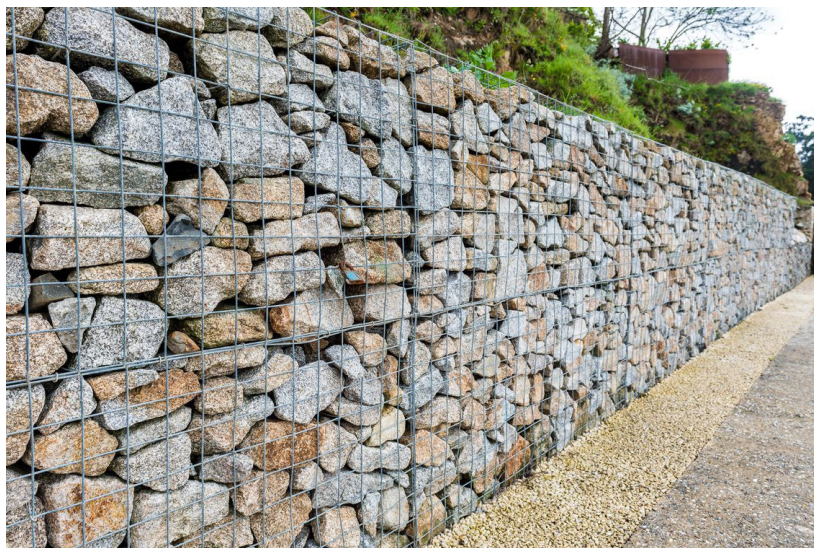
A gabion wall is an affordable way to make a dramatic visual statement
